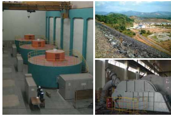
ユンカン発電所の発電機(左)、ビリビリ発電所のダム外観(右上)、及びダニム発電所の水車(右下) Generators for Yuncan Power Station (left), dam site for Bili Bili Power Station (top right), and turbine for Da Nhim Power Station (bottom right)
