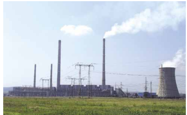
View of turbine building
