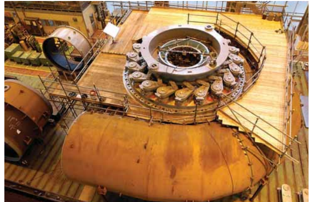
Shop assembly of pump-turbine for Purulia Pumped Storage Plant
