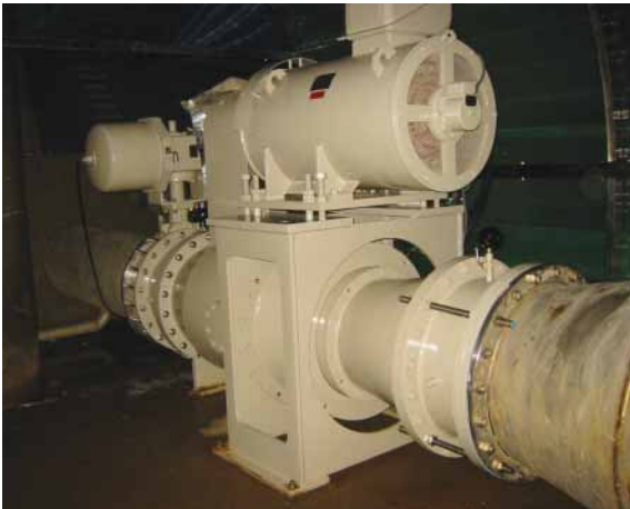
Micro hydro power generating equipment for sewage treatment plant in Taichung Science-Based Industrial Park
