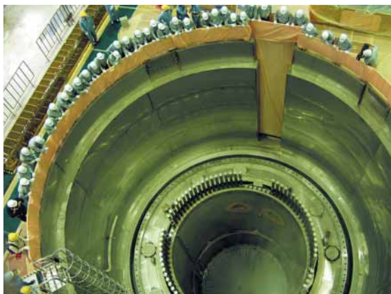
東北電力(株)東通原子力発電所1号機のECCS注水試験 Emergency core cooling system (ECCS) spray test at Higashidori Nuclear Power Station Unit No. 1 (1,100 MWe, BWR) of Tohoku Electric Power Co., Inc.
