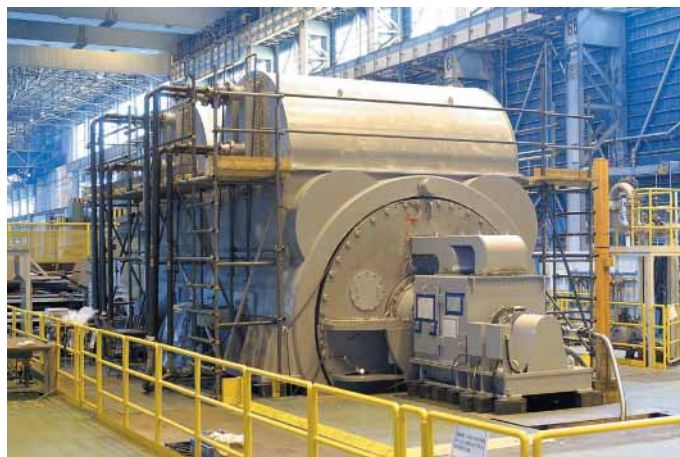
大容量空気冷却発電機の工場回転試験 Rotating shop test of large-capacity air-cooled generator
