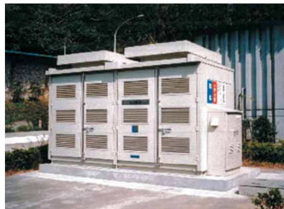
250 kW NaS 電池 250 kW NaS battery for energy storage system
