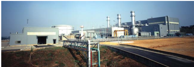
Chiahui Power Station, Taiwan
