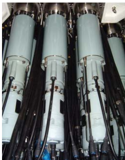
View of installed S-FMCRD
