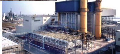
Chang Bin Power Station, Taiwan
