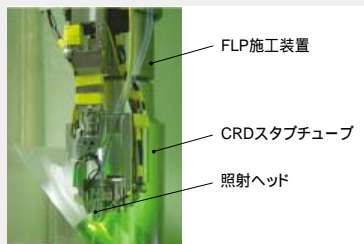
炉底部FLP施工装置 Fiber laser peening equipment
