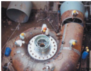
The spiral casing at Sipansihaporas Power Station (1×17.6 MW, November 2002), Indonesia
