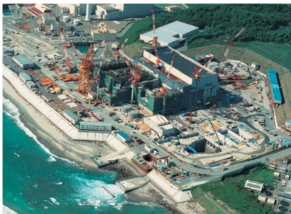
中部電力(株)浜岡原子力発電所5号機 1,380 MWe, ABWR) Hamaoka Nuclear Power Station Unit No. 5 of Chubu Electric Power Co., Inc. (1,380 MWe, ABWR)
