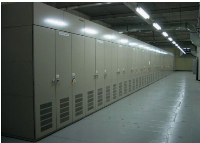
50 Hz/ 60 Hz静止形周波数変換装置 50 Hz/ 60 Hz static frequency converter
