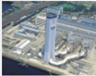
Shinagawa Thermal Power Station of The Tokyo Electric Power Co., Inc.
