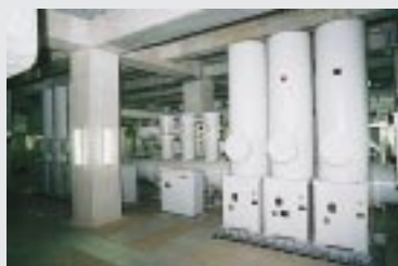
東京電力(株)新豊洲変電所向け550 kVガス絶縁開閉装置 550 kV gas-insulated switchgear for Shin-Toyosu Substation of The Tokyo Electric Power Co., Inc
