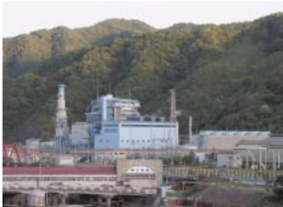
新日本製鐵(株)棒線事業部 釜石製鐵所発電設備全景 Overview of Kamaishi Works Thermal Power Station operated by Bar & Wire Rod Div. of Nippon Steel Corporation
