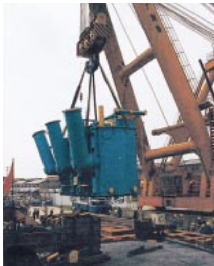
CTC埠頭での750 MVA変圧器の船積み Shipping of 750 MVA transformer at CTC Wharf
