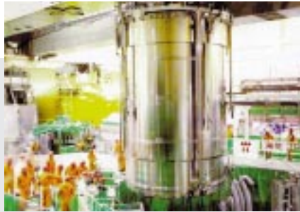
Installation of core shroud into reactor pressure vessel
