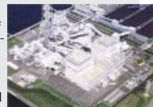
Nanao-Ohta Thermal Power Station of the Hokuriku Electric Power Co., Inc.
