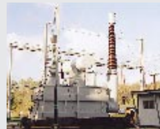
250MVA-500/√3 kV large capacity, high voltage single-phase oil-immersed transformer
