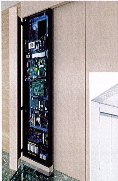
SPACEL™制御盤 Control panel of SPACEL™ machine-roomless elevator
