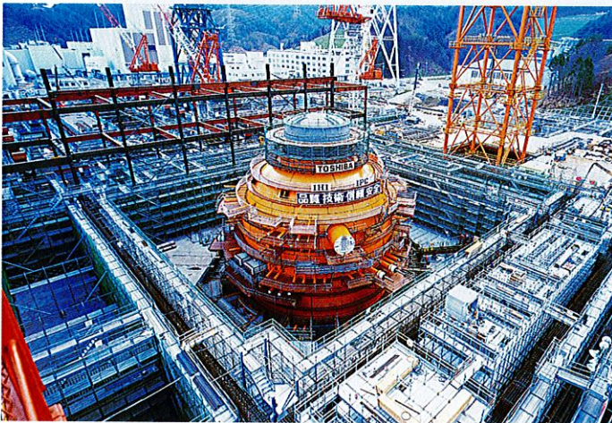
東北電力(株)女川原子力発電所3号機(825 MWe, BWR-5) Onagawa Nuclear Power Station Unit No. 3 of Tohoku Electric Power Co., Inc. (825 MWe, BWR-5)
