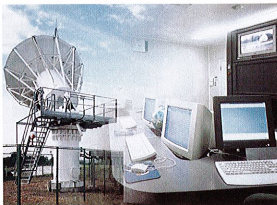
空中線と監視室 Antenna and monitoring center
