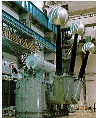
360MVA-500kV step-up transformer for An Shun Power Station
