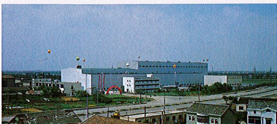
Changzhou Toshiba Transformer Co., Ltd.
