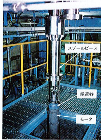
改良型 FMCRD Advanced fine-motion control rod drive
