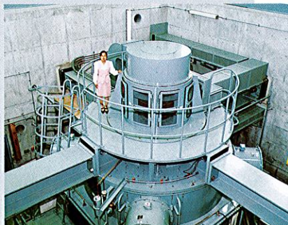
Adjustable-speed flywheel generator
