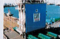
Off-loading of heat-recovery steam generator (HRSG)
