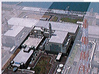
Kashiwazaki-Kariwa Nuclear Power Station Unit No. 6 of The Tokyo Electric Power Co., Inc.
