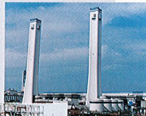
Yokohama Group 7 and 8 power plants of The Tokyo Electric Power Co., Inc.
