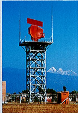
Radar site building and radar antenna
