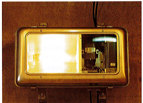
光触媒膜付きトンネル照明器具 Tunnel luminaire with photocatalytic thin-film-coated glass
