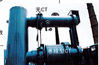
光ファイバ電流センサと原理 Optical current transformer and its principle
