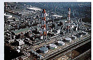
Aerial view of Chita Thermal Power Station (Units No. 1-6)
