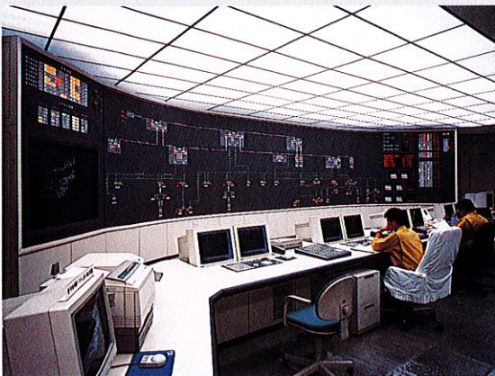
Operation room of central dispatch center
