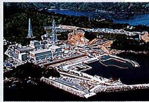
Onagawa Nuclear Power Station Unit No. 2 of Tohoku Electric Power Co., Inc.
