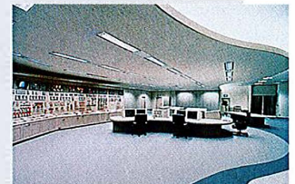
Central control room at Reihoku No. 1 unit
