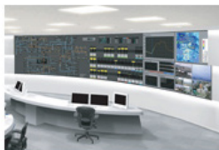
Supervisory Control And Data Acquisition Systems (SCADA)
