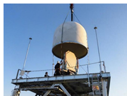
MP-PAWR at time of installation at Saitama University (before covering the antenna with a radome)
