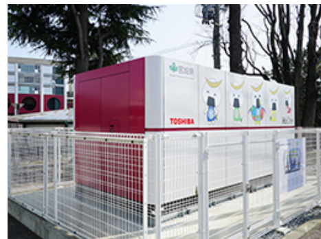
H2One™, Hydrogen energy supply system for Rakuten Seimei Park Miyagi
