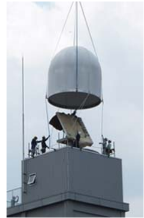
Weather radar being constructed
