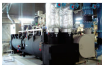
State-of-the-art high efficiency inverter centrifugal chiller
