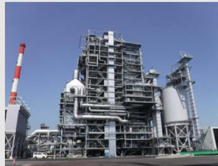
Mikawa Biomass Power Plant
