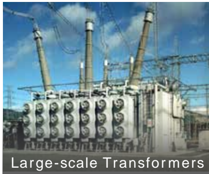
Power transmission and distribution (T&D)
