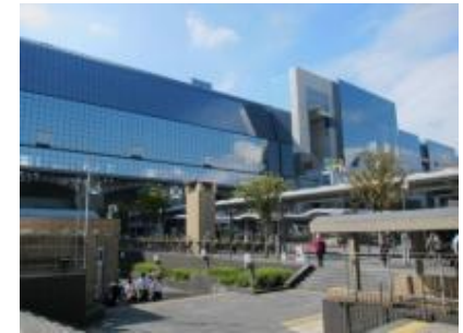
Station building heat source equipment replacement (Kyoto) 28 units chiller
