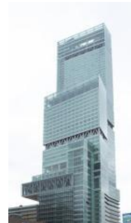
Abeno Harukasu Tallest high-rise building in Jaapan 29 elevators installed (Including 22 high speed elevators)
