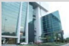
UEM India Pvt. Ltd. Water treatment systems (EPC*)
