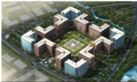
"Hangzhou Bafang Castle City Comprehensive System" (China) 3,790 units Multi-air-conditioning unit
