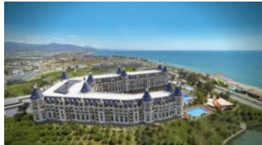
HAYDARPAŞA PALACE HOTEL (Turkey) 180 units Multi-air-conditioning unit
