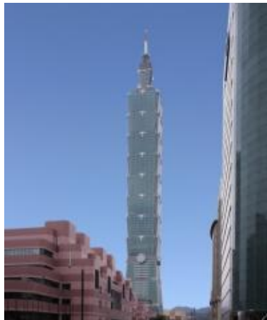
Taipei 101 World's fastest class high speed elevator 12-year accident free operation 61 elevators installed (Including 2 ultra high speed elevators)
