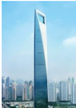
Shanghai World Financial Center 11 elevators installed (3 ultra-high speed elevators and 8 double deck elevators)
