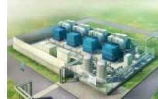
A fuel cell power plant running on ADG*5
