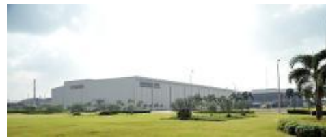
Toshiba JSW Power Systems Private Ltd. (India)
