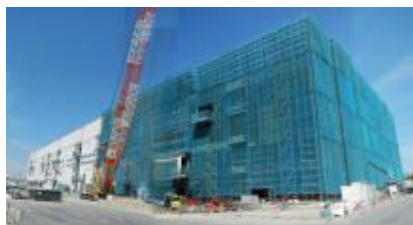
2 nd phase of construction of Fab No. 5 in Yokkaichi
