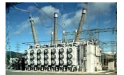
Advanced site-assembly three-phase transformers
