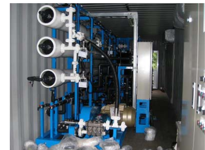
Seawater desalination system
