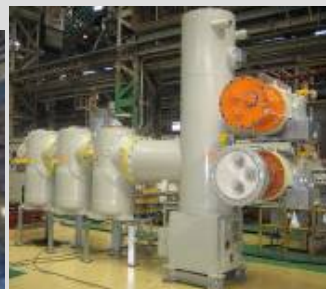
Compact type 145kV GIS in world's smallest class
