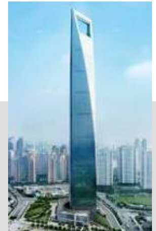
Shanghai World Financial Center 600 meters a minute, the fastest* elevators in mainland China (*Source: Toshiba)
