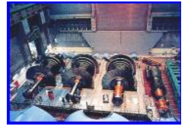
Inspection of Turbines
