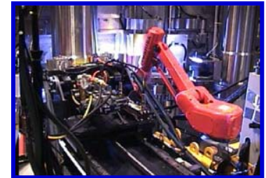
Full Automatic Welding Robot in Reactor
