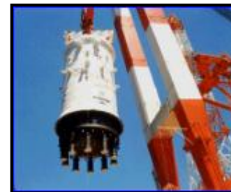
Installation of Nuclear Pressure Vessel
