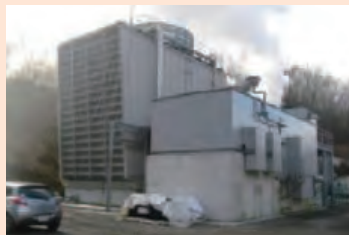
Waita Geothermal Power Plant
