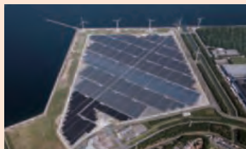
Tahara Solar - Wind Joint Project Tahara Solar/Wind Electricity Generation Plant (50MW)
