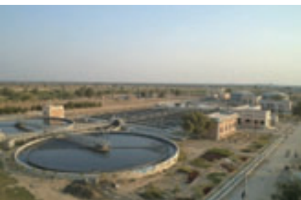
A water sewage treatment plant in India constructed by UEM
