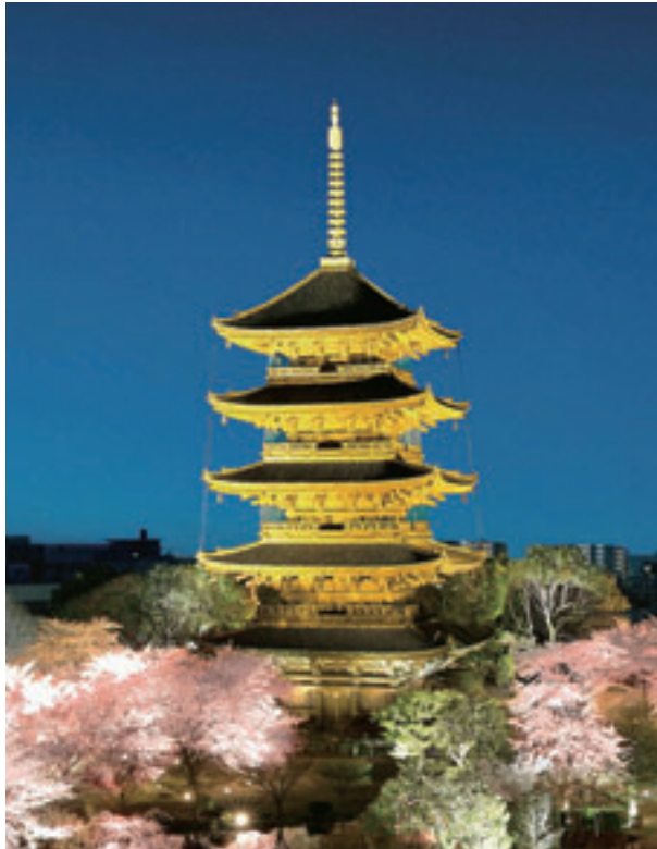
The "golden five-story pagoda" of Toji Temple in Kyoto, lit up with LED lighting
