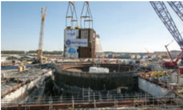
©2014 Georgia Power Company All rights reserved Installation of the largest module of the AP1000™, under construction in the US
