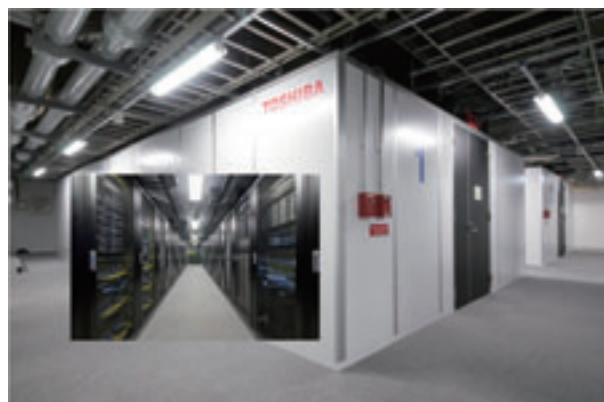
Cloud & Solutions Company, Data Center Image
