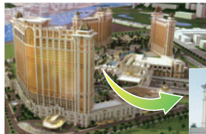
Order won for 209 elevators at the Galaxy Hotel under construction in Macau (first and second phase total)
