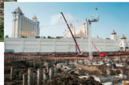
(second phase is currently under construction)
