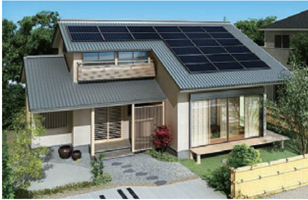
Residential solar power system
