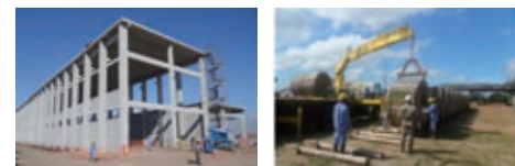
Toshiba Infrastructure Systems South America Ltd. Construction in progress in the plant Toshiba won
