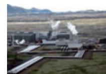
Geothermal power plant installed by Toshiba
