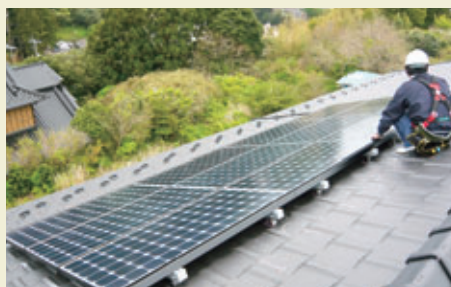
Donated photovoltaic power generation systems to 18 facilities, such as rescue shelters
