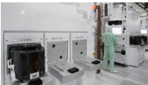
Fab 5 at Yokkaichi Operations (Clean room)
