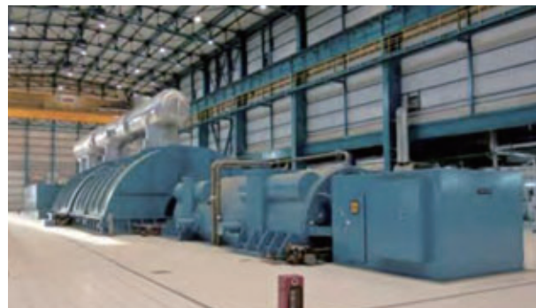
Tanjung Jati B Coal Fired Power Plant in Indonesia at 660 MW steam turbine generator
