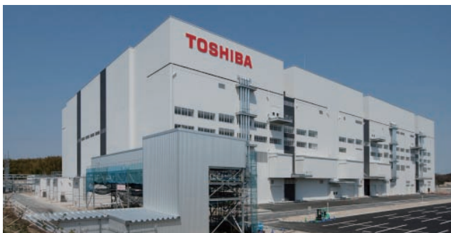
Yokkaichi Operations has completed construction of its Fab No.5 wafer production facility. Production started in July 2011.
