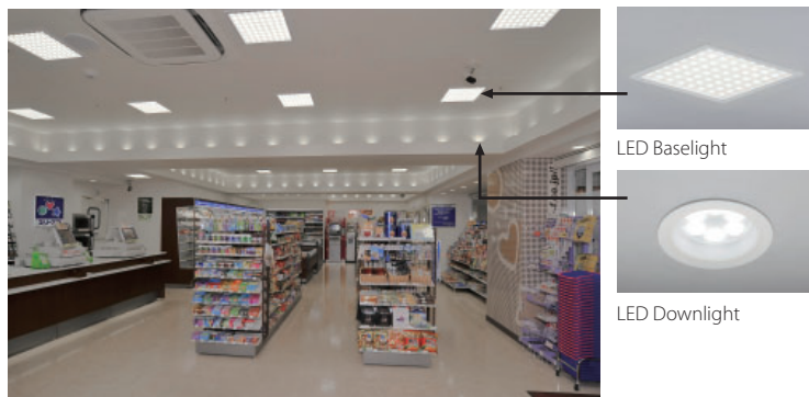
A convenience store lit with LED lighting (Three-F store in Yokohama City Government Office)
