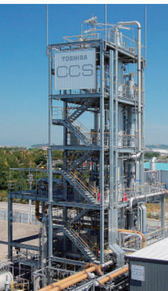
Pilot plant CO 2 separation and capture plant, (Sigma Power Ariake Co. Ltd.'s Mikawa Power Plant)
