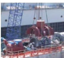
Toshiba's No.3 position in the 2001 global market for steam turbines has recently been strengthened by supply of equipment to many thermal power plants in North America.
