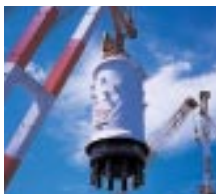
Chubu Electric Power Co., Ltd.'s No. 5 Unit at Hamaoka Power Station, currently under construction, integrates Toshiba's most advanced ABWR. (Picture: Installation of nuclear reactor vessel)
