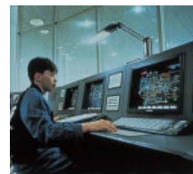
Toshiba's production monitoring and control system for a brewing company realizes an open, streamlined system. Close integration with the host system realizes real-time process management.
