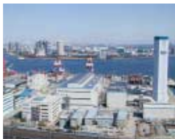
Toshiba is the main contractor for the 1140MW substation at TEPCO's Shinagawa No. 1 Thermal Power Station. This 1300°C gas turbine combined-cycle power plant is scheduled to commence operation in July 2001.
