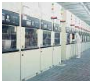
The clean room at Oita Operations produces system LSIs for digital consumer equipment, networks and communications equipment. A new annex, opened in April 2001, has expanded operating scale and technological capabilities.
