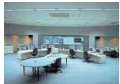
State-of-the-art monitoring and control systems improve reliability for this water-treatment system. An ergonomic design for the monitoring room itself ensures a comfortable, operator-centered work environment.
