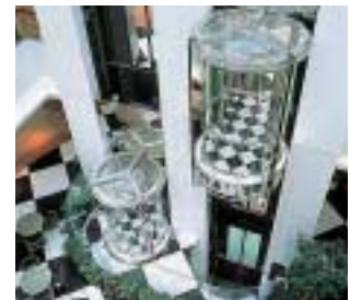
Toshiba's keen attention to design is clear to see in these elevators in a Singapore shopping center.
