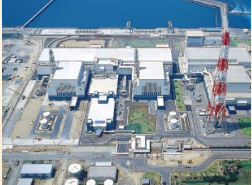
In fiscal 1997, Unit No. 7 at TEPCO's Kashiwazaki-Kariwa Nuclear Power Station started commercial operations.
