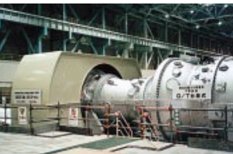
The Shin-Nagoya Thermal Power Station uses a highly efficient Toshiba combined-cycle generation system.
