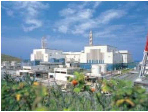
Commercial operation of the world's first ABWR began in 1996 at Unit No. 6 of Kashiwazaki-Kariwa Nuclear Power Station. The unit was built by a consortium led by Toshiba and incorporates many technological advances.
