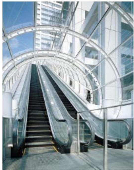
Attractive Toshiba elevators and escalators are integral elements of the striking new Tokyo head office building of Fuji Television Network.
