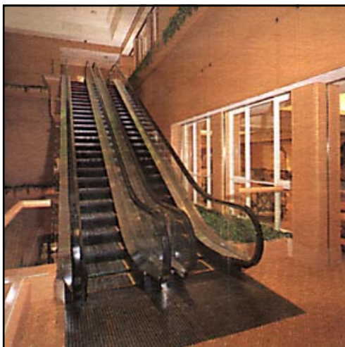
Toshiba elevators and escalators, like these in the Hotel Intercontinental Tokyo Bay, offer a smooth, reliable ride.
