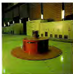
Toshiba generating equipment is a key element of the Chaira pumped storage power plant in Bulgaria. The plant's 701-meter pumping head is the world's highest.
