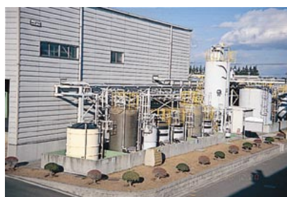
Dikes for tanks containing liquid chemicals
