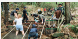
Constructing a check dam over the stream in the forest
