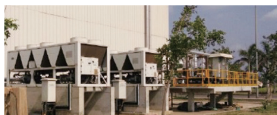
Raising the floor of equipment in preparation for disasters
