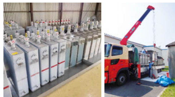
PCB-containing equipment being transported to JESCO
