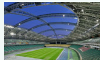
Floodlights installed in Oita Bank Dome
